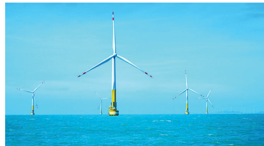
The Pinghai bay offshore wind power project in Putian, southeast China's Fujian Province. (PHOTO: XINHUA)
