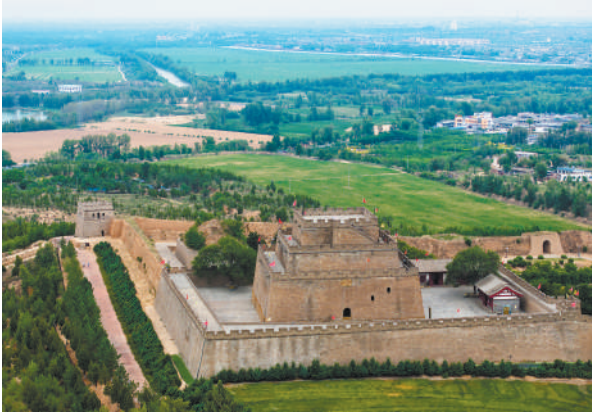
The "Zhenbeitai" watchtower in Yulin, northwest China's Shaanxi province. Yulin has positioned itself to play an important role in China's energy transition. (PHOTO: XINHUA)
