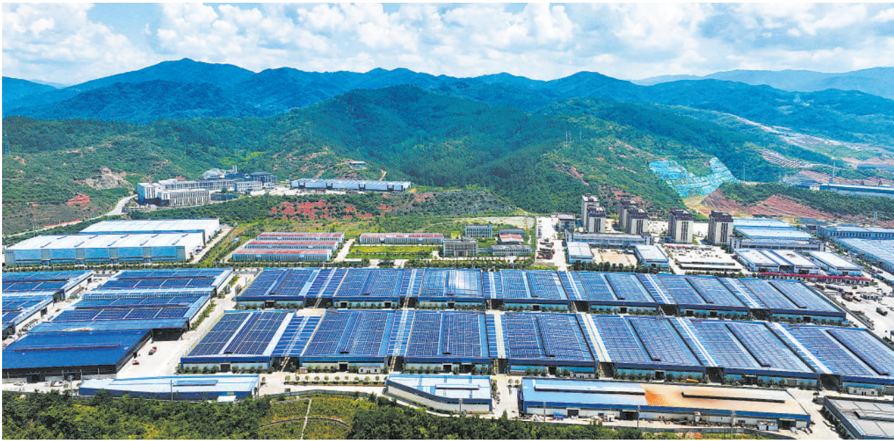
Fangxian county in Central China's Hubei province gives full play to its solar energy resources and taps idle factory rooftops to build photovoltaic projects in industrial parks, June 29, 2026. (PHOTO: VCG)
